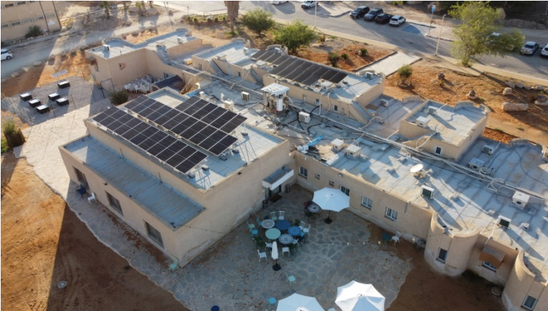
Solar system that heats water on the spot and produces electricity.
