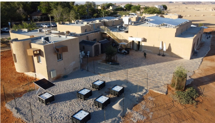
Hydroponic system with one solar panel only.
